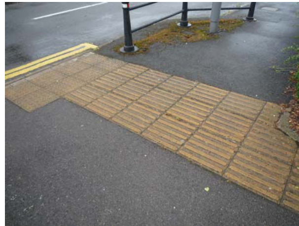
Blister paving and guidance paving used at crossing points along High St
