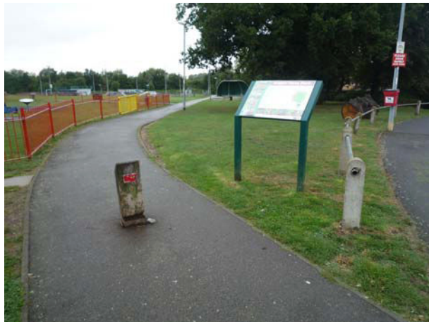
Example of low level bollard in path and information panel which cannot be read by anyone seated or short of stature.
