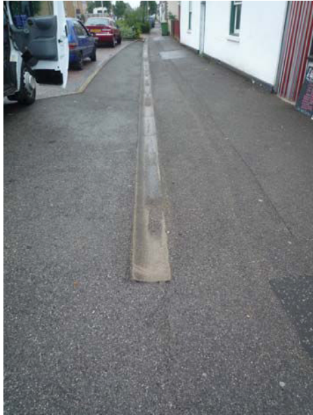
Dished gully used in the middle of the footway
