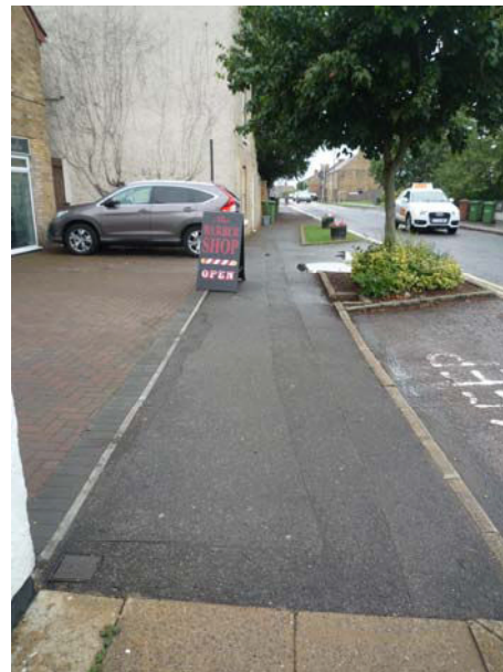
Blister paving and guidance paving used at crossing points along High St
