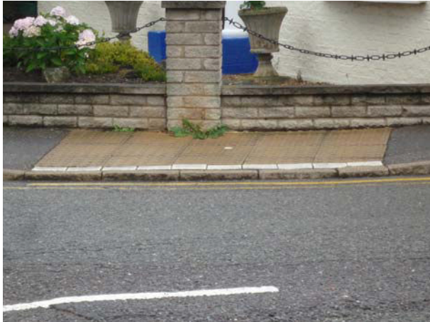
Dropped kerb at the roundabout at the end of Thorney Rd
