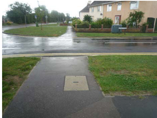
Little Close with a dropped kerb but no blister tactile warning
