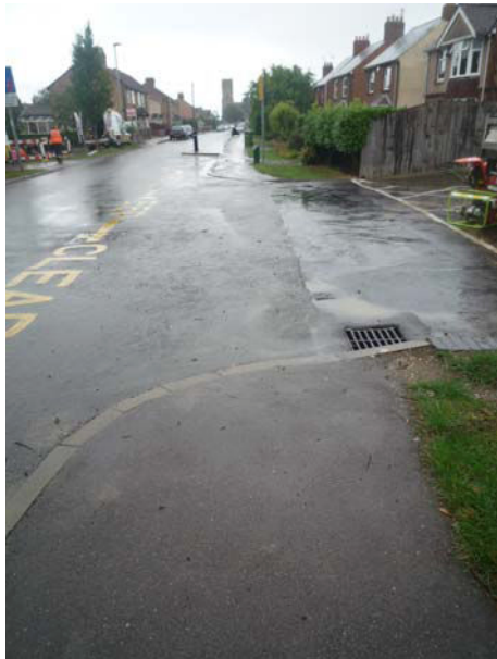
Vehicle crossover to the school, no tactile warning
