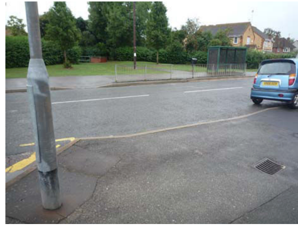
Dropped kerbs adjacent to the bus stop and roundabout with High St
