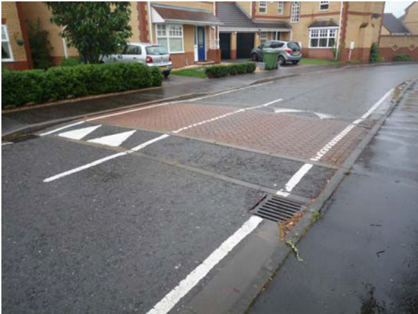
Raised carriage way makes a good crossing point but not flush with kerb and no blister warning
